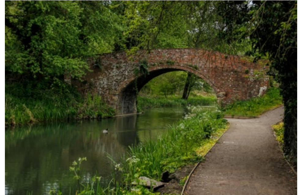
Image 53 Footpath on the Severn Thames Canal
