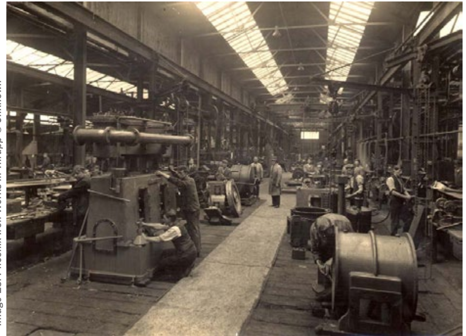
Phoenix Iron Works at Phoenix Mill, run by Geroge Waller in the 1870's.
