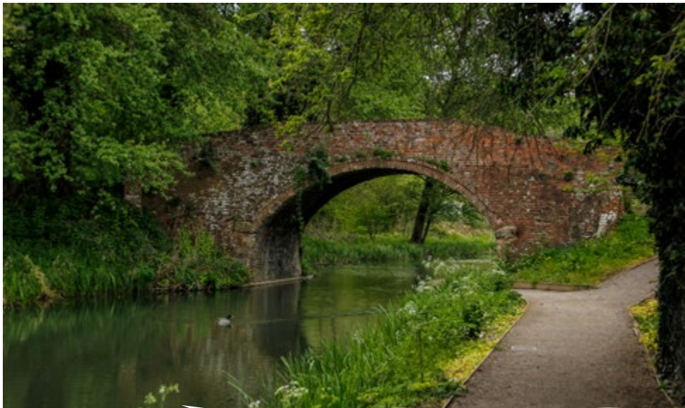
Image 30: Bridge over Severn Thames Canal
